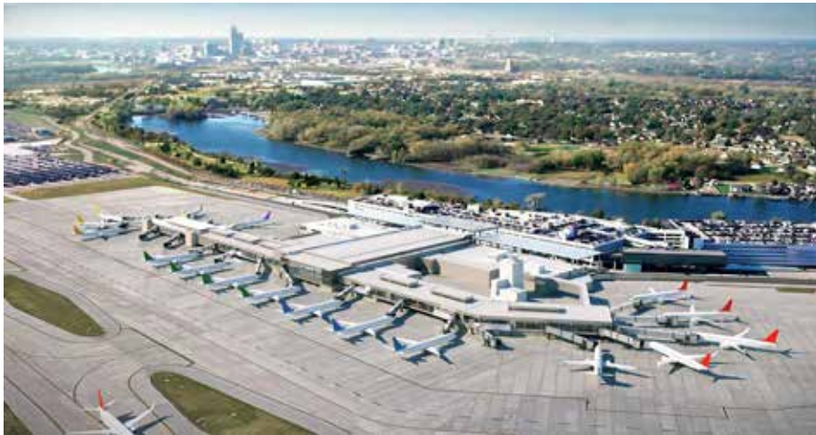
Pic4 – Omaha Eppley Terminal Modernization
