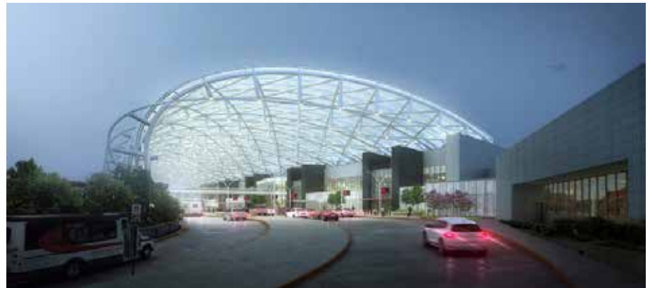
Pic1 – Curb side Canopies – Hartsfield Jackson International Airport
